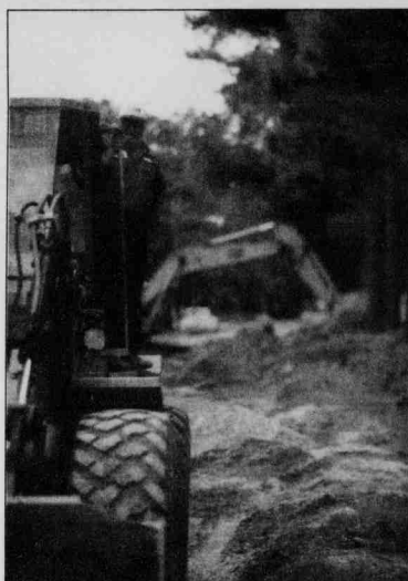
(middle) Construction in front of D.H. Library has closed off passage between the buildings and Hillsborough Street. (bottom) Sullivan Drive should be repaved by August.
