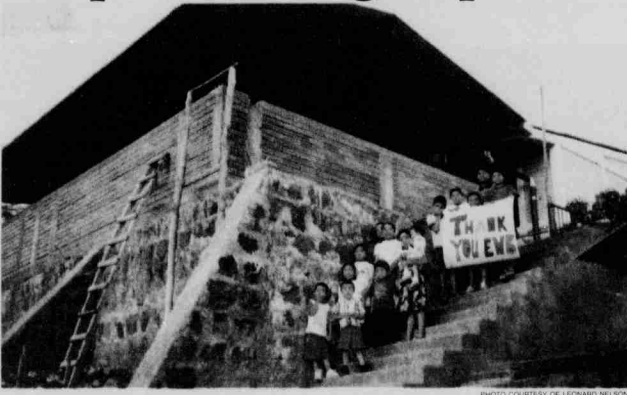
NCSU's Engineers Without Borders had planned to wire this El Salvador school for electricity, but the country's Jan. 14 earthquake may have damaged or destroyed the school.
