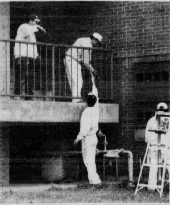
Painters work to paint over lead-based paint from the railings at the E.S. King Village.
