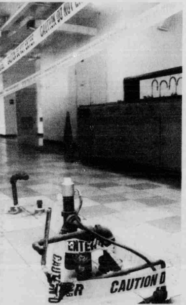
If the bond referendum passes Nov. 7, NCSU could receive $468 million for the renovation and repair of such facilities as this Withers Hall laboratory.
