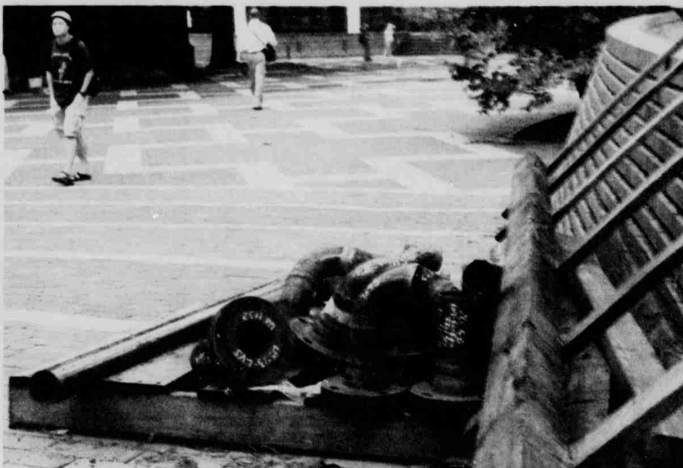
Construction work around Harrelson Hall continues at a feverish pace, causing students slight detours. These bricks will likely be bruised and scuffed badly by the heavy equipment. We anticipate that new bricks will soon take their place.
