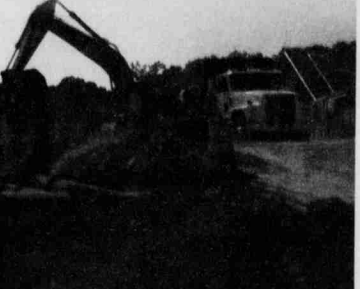
Constant construction has been the theme this summer. (Top) Sidewalk construction on Cates Avenue create a pedestrian detour on the street, causing orientation traffic of all types to compromise. (right three, bottom) Centennial Campus development.
