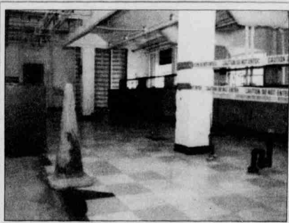
One of the labs in Clark hall currently under renovation.
