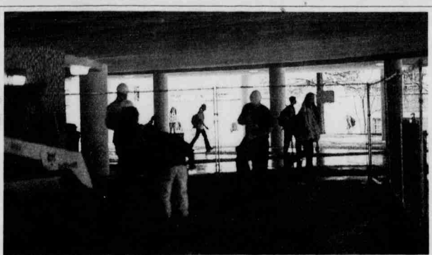
Students are forced to walk around a fenced area under Harrelson while workers do their thing.
