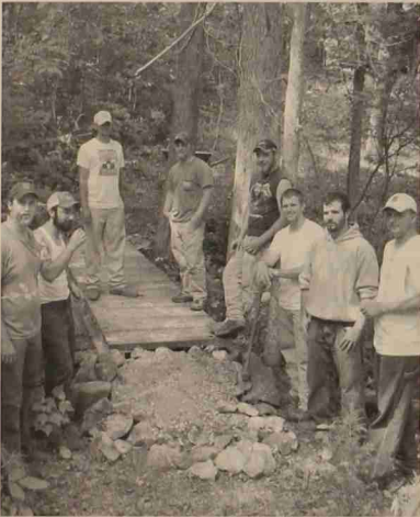
FOR 273 students placing and securing a bridge over a swampy area.
