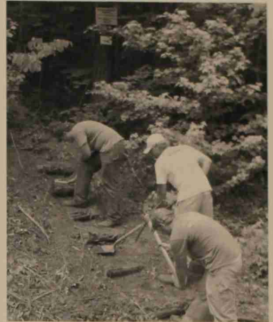
FOR 273 students repairing stairs on a commonly used trail.
