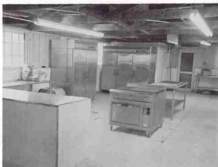
Remodeled kitchen at Slocum Camp.
