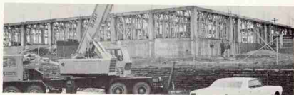
The new School of Forest Resources building. (Under Construction)
