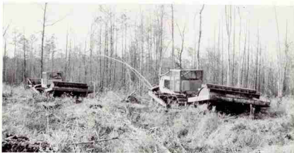
Site preparation for planting. The drum chopper begins the process that will start the new forest. N.C.F.S. Photo
