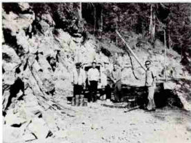
Forest Service road construction.
