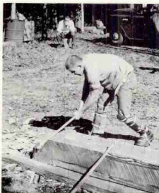
Chandler Eakes puts the steel to the wood!
