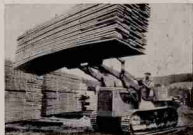
Tractor shovels with attachments for loading and handling logs and finished lumber, handling variety of maintenance jobs in the woods or at the mill.
