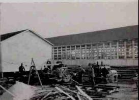
Woodshop and Saw Mill
