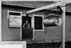
Track arranged with slight Incline so carrier may be emptied with trip rope and returned to barn. A barn in Sweden.
