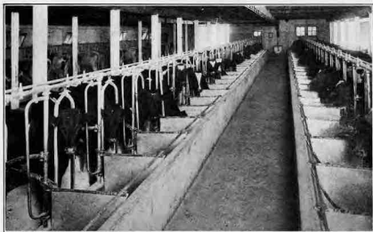
Louden Stalls, Stanchions and Manger Divisions in the Haskell Institute Dairy Barn
