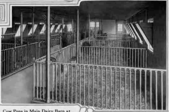
Cow Pens in Main Dairy Barn at Homewood Farms, Louden planned and equipped
