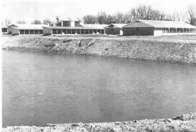
Settling ponds or lagoons, like this one at the dairy facility on the Piedmont Research Station, became a useful tool in the handling of animal wastes.
