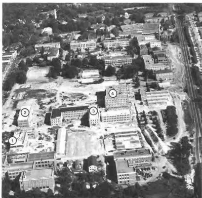
Four agricultural buildings, under construction in 1951, are shown in this aerial photograph of the campus looking east: (1) Kilgore Hall (Horticulture and Forestry), (2) Scott Hall (Poultry Science), (3) Gardner Hall (Biological Science), (4) Williams Hall (Agronomy). Note area cleared for construction of the first student union building and D. H. Hill library in upper left corner.
