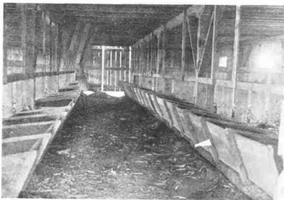
Interior of the cattle barn at the Iredell Test Farm.
