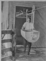
Fig. 1287—Using the Louden Self-Acting Carrier on the Louden Combination Steel and Rod Track
