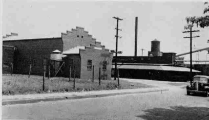
THIS GIN, OPERATED IN CONNECTION WITH A COTTON OIL MILL, IS A PERMANENT BRICK BUILDING.
