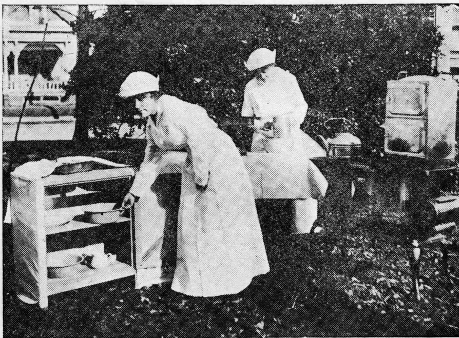
PREPARING FOR THE DEMONSTRATION
