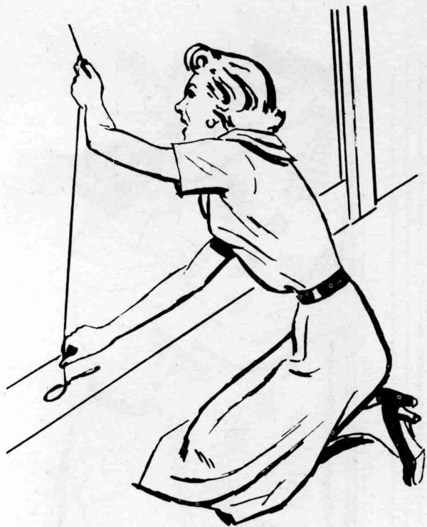
2. Use a plumb line to get first strip of paper straight.
