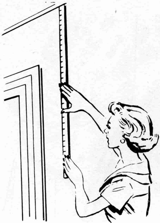
1. To figure length of first strip, measure wall with yardstick.
