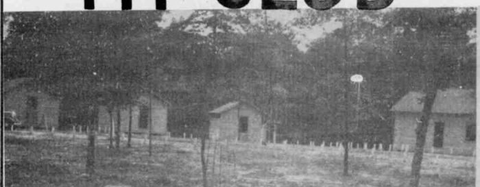
Completed Cottages at 4-H Club Camp In Bertie County.
