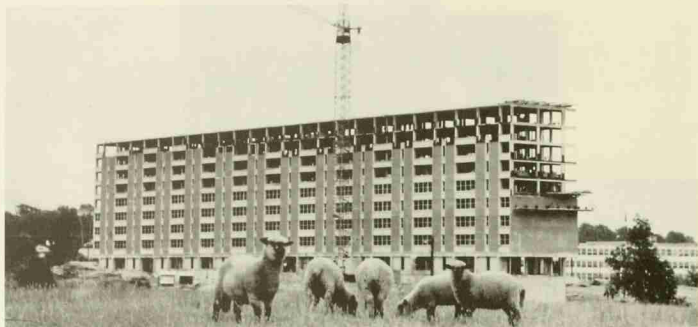
Construction of Lee Residence Hall. Vol. 62
