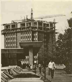
Construction of the Tri-towers. Vol. 66 BELOW
