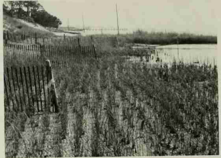
struction of concrete walls. Protective vegetation shrouds the same scene five months later (right).
