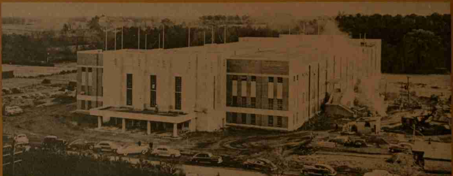
Reynolds Coliseum under construction, 1949.
