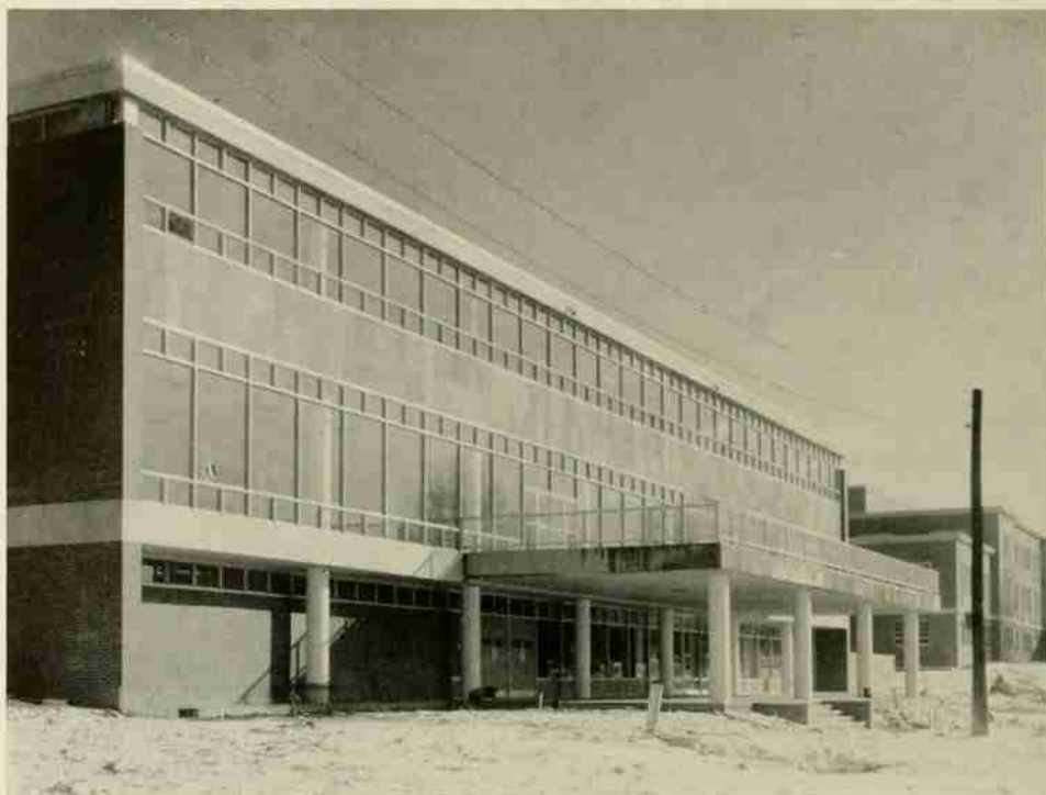
college union building nears completion
