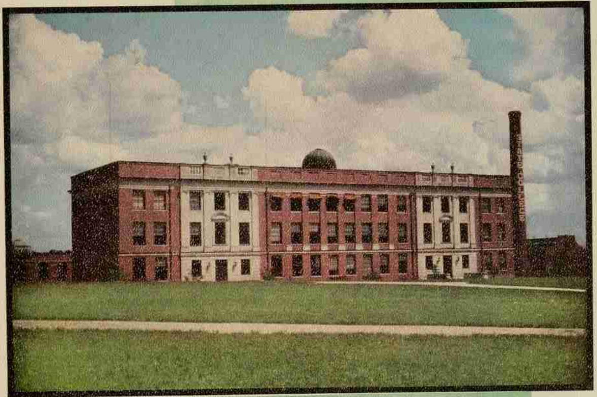
DANIELS HALL. Departments of Physics and Electrical Engineering
