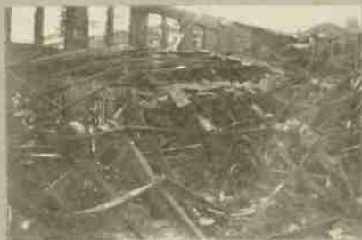
BEFORE AND AFTER THE FIRE
