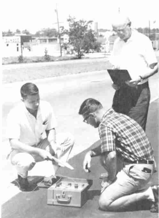
Chemical engineering and civil engineering graduate students and faculty cooperate on highway research. Recording temperature measurements of test strips on a North Carolina highway is part of the bituminous highway project.
