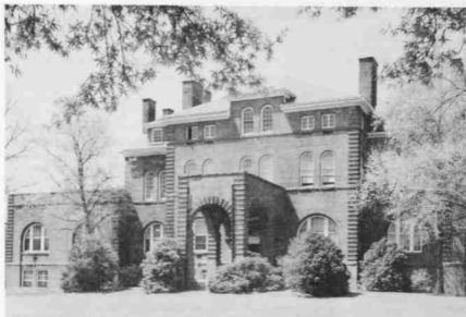
Holladay Hall is the oldest building on the State College campus.
